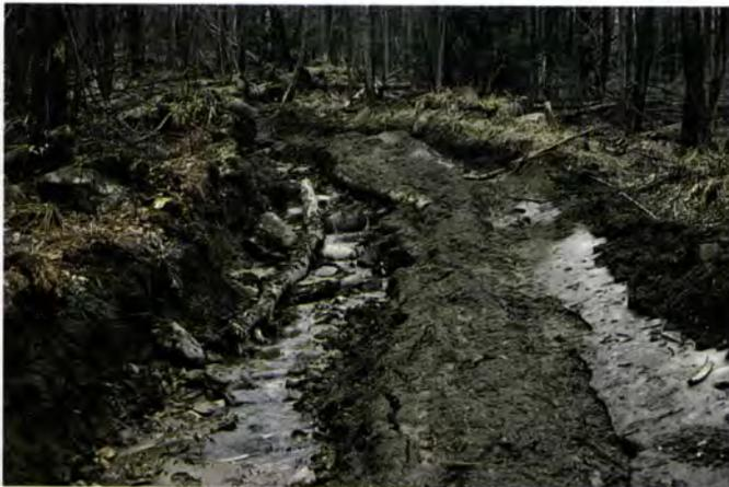
*Use of wet roads results in ruts, which can lead to erosion on roads that are neglected or poorly maintained. Improperly used roads are rough on the eyes and the land, as well as the contractor's equipment, pocketbook, and reputation.*
