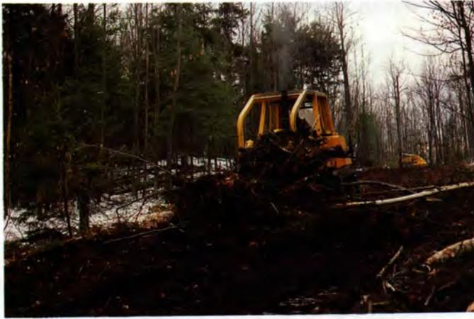
*The negative impact of truck road construction can be reduced by cutting trees before bulldozing. Remove merchantable sections of wood and bury or push aside unmerchantable wood and debris.*
