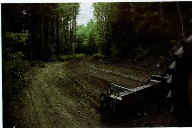
*Ditch, crown, and grade roads after use to reduce erosion and leave a more positive sense of stewardship.*
