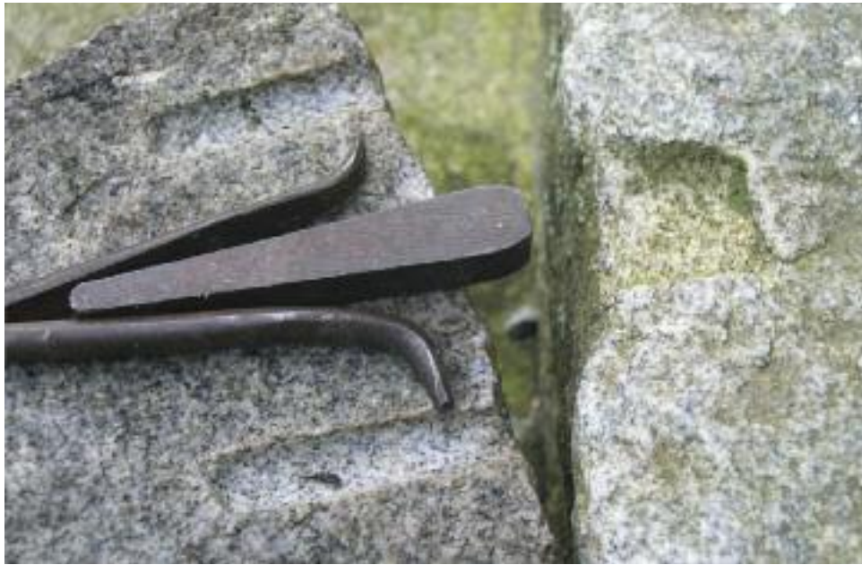
On left, a thick steel wedge lies between the two thin “feathers” on a block of granite split after 1840 as evidenced by round bore holes drilled with a star bit on a plug drill. On right, the rectangular signature of a square chisel from a stone quarried and split prior to 1840.
