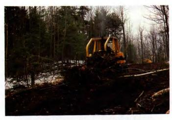
The negative impact of truck road construction can be reduced by cutting trees before bulldozing. Remove merchantable sections of wood and bury or push aside unmerchantable wood and debris.
