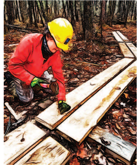
Trail crew volunteer Beth Sullivan of Billerica, Mass., works on a bog bridge at Powder Major's Forest.
