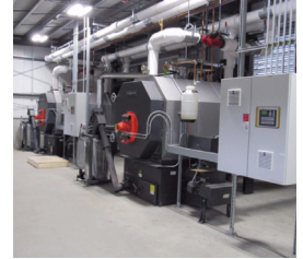
A biomass thermal system can provide hot air, water, and process heat
