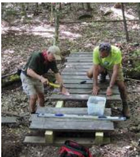
Terry Irwin (left) and Len Martin (right) construct a trail footbridge on the Buxton-Simons Forest in Weare.
